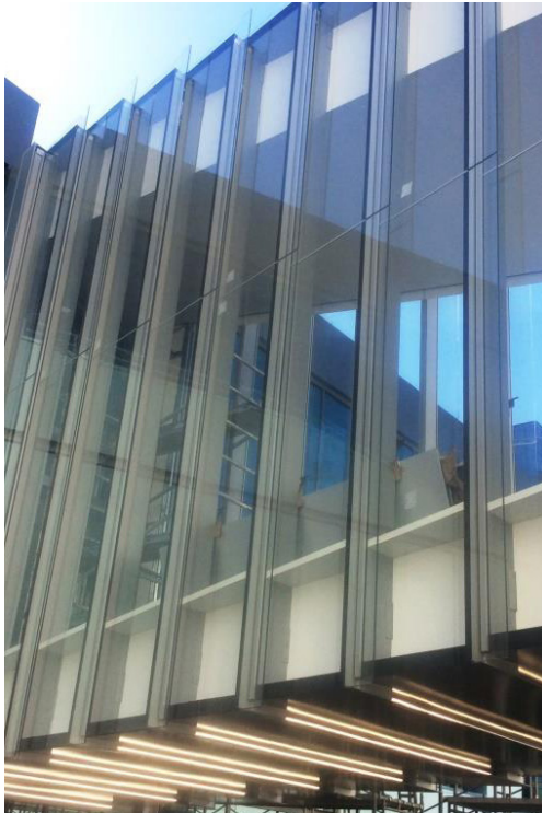
Twitter Skybridge Bohlin Cywinski Jackson Custom Unitized Curtainwall
