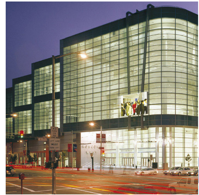
Moscone Center HOK Group, Inc. SuperWall™ and Custom Unitized Curtainwall
