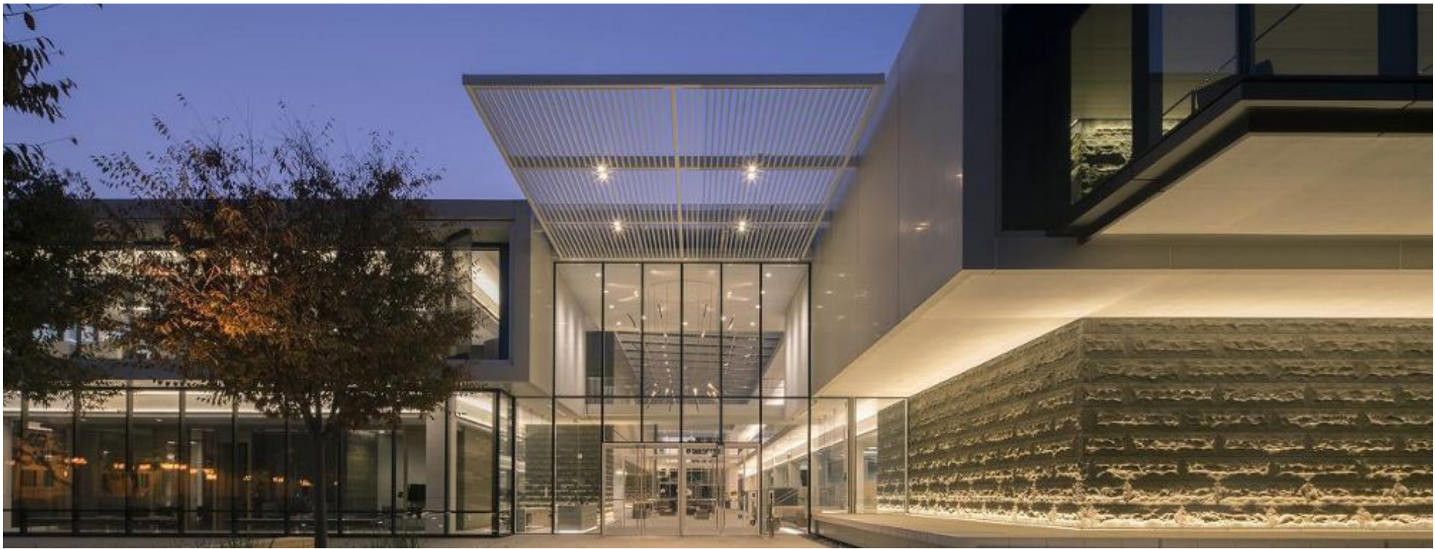
E&J Gallo Winery Gensler SuperWall™ and SSG
